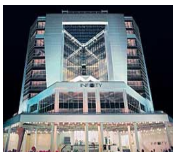
An IT building in Sector V
