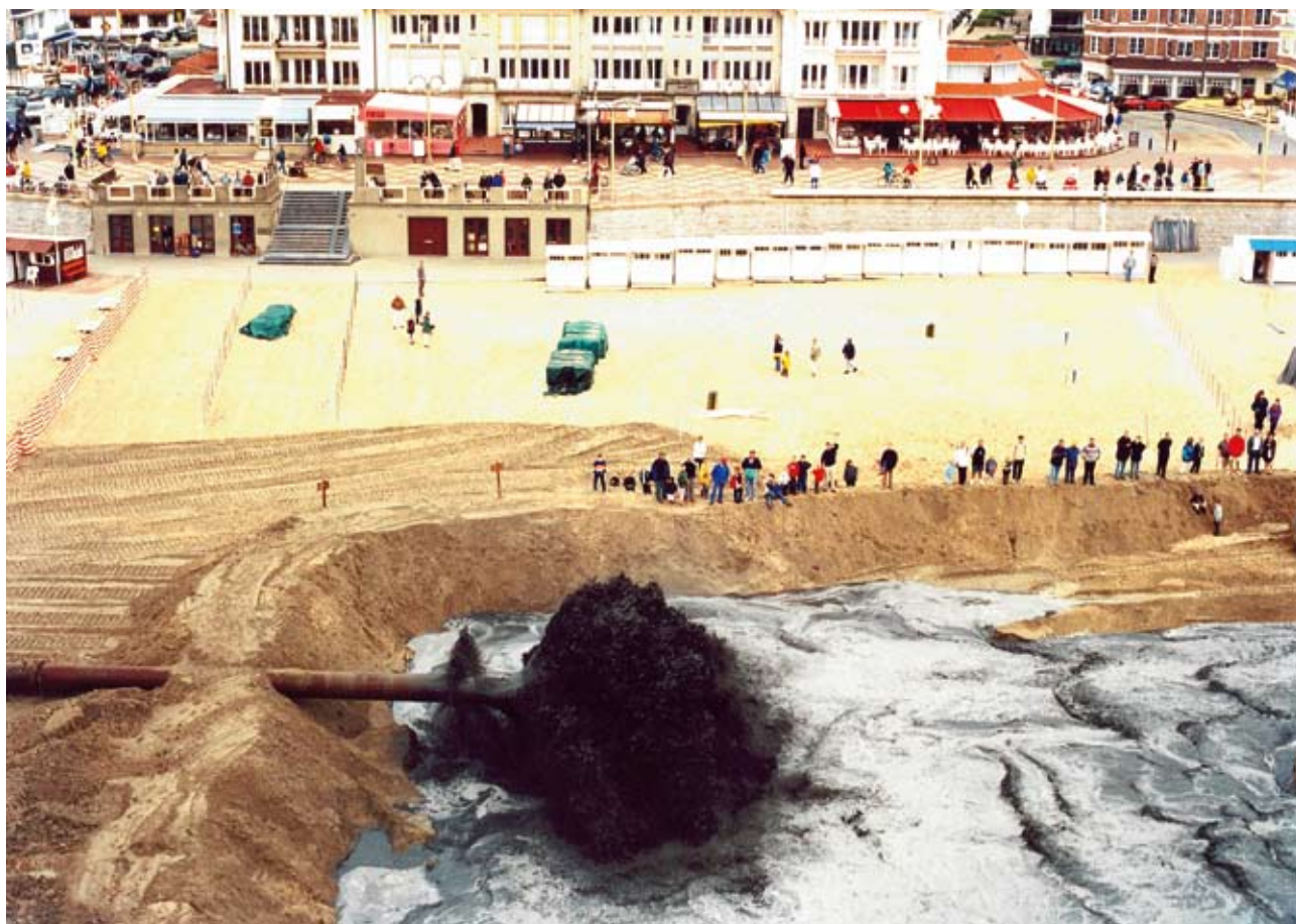
Tonnes of sand are pumped onto the beach at De Haan to shore up defences
