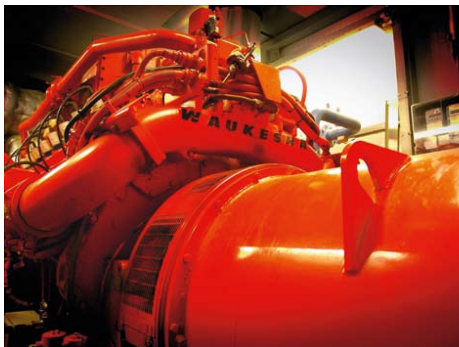
The specially made engine that pumps the power from farm source to holiday park itself operates on a mix of methanes and bio-fuel
