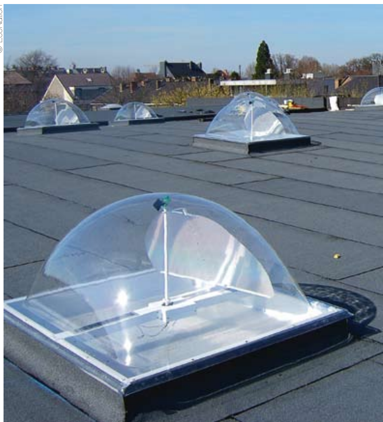
The roof-top LightCatcher spreads light throughout a building without the use of electricity
