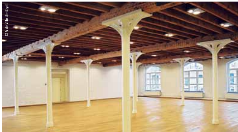
The interior of De Markten, built following an English design that protected mills from fire
